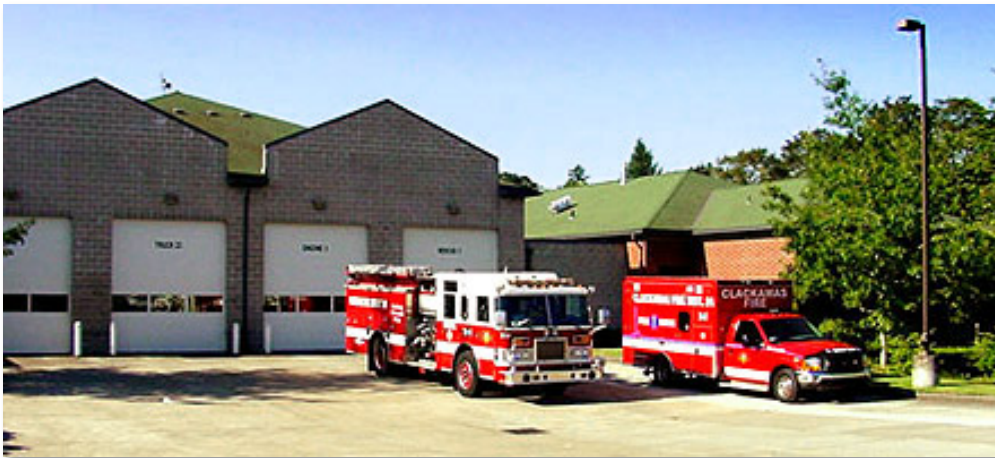
Exterior View at apparatus bays
