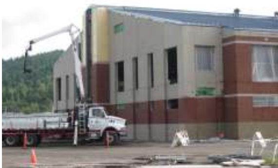
West End of Building Under Construction
