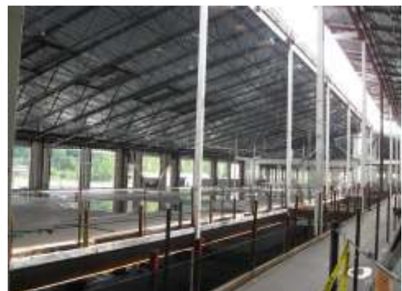
Second Level Office Area Under Construction
